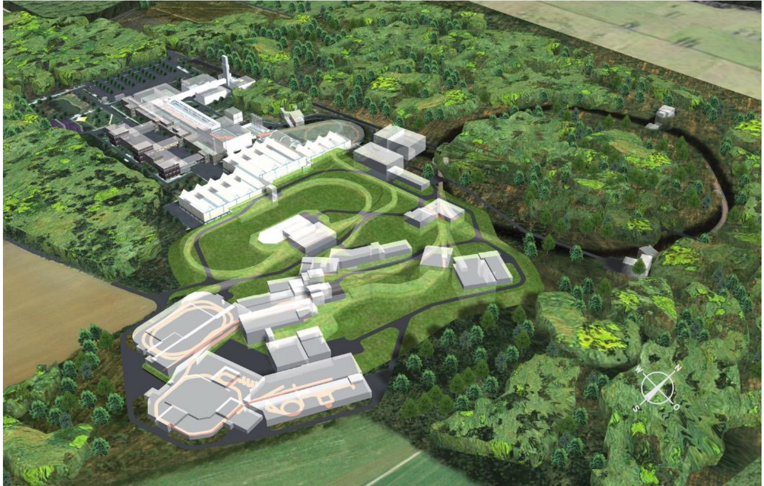
Figure 1.1: Artists view of FAIR. The synchrotrons on the right will be located 10 to 13 m underground and will not be visible in reality. Most of the roofs will be vegetated and thus most of the facility will be hidden from view.
